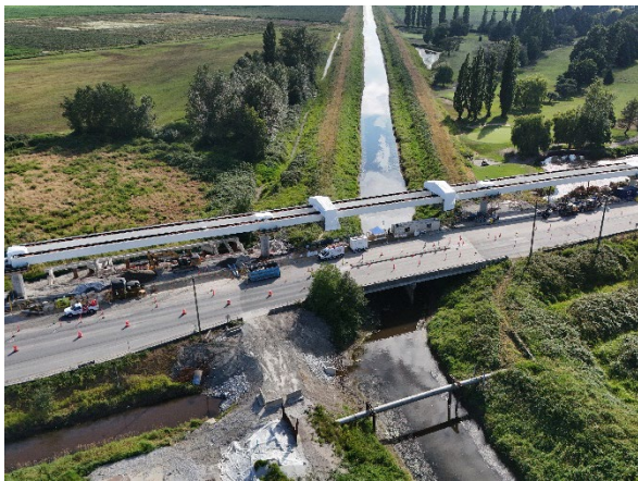
Figure 3: Steel beams installed over the Serpentine River west of Highway 15.
