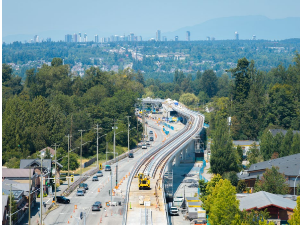
Figure 1: Completed guideway west of 68 Avenue, marking the milestone of 50% guideway completion.
