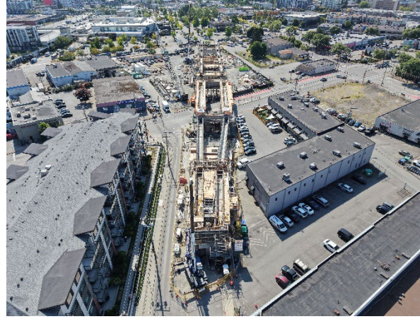
Figure 2: Guideway beams installed at east end of Industrial Avenue.
