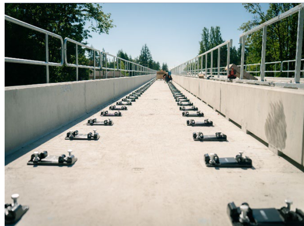
Figure 4: Section of rail mounting plates installed near 148 Street.
