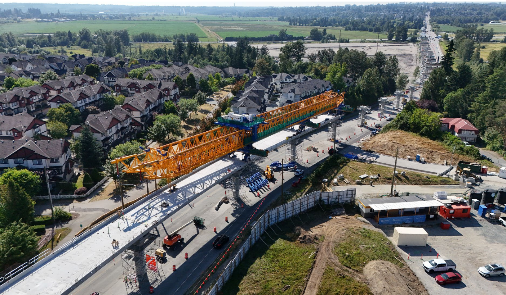
The Clayton Clipper installs elevated guideway segments.
