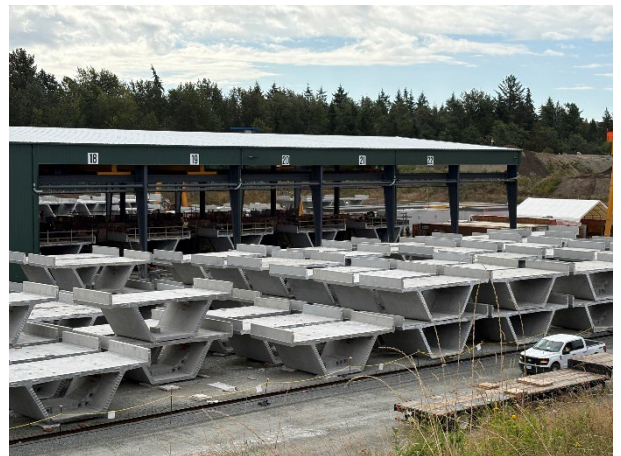
Concrete segments stored at the precast yard.
