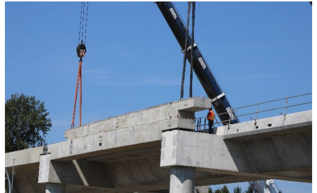
Beam installation at 152 Street Station.
