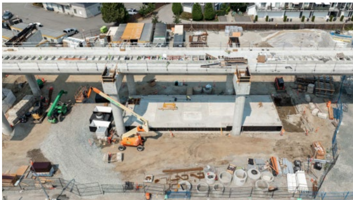
Station construction at the future 152 Street Station.
