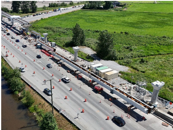
Figure 3: Steel beams staged west of Highway 15, ready for upcoming guideway installation.
