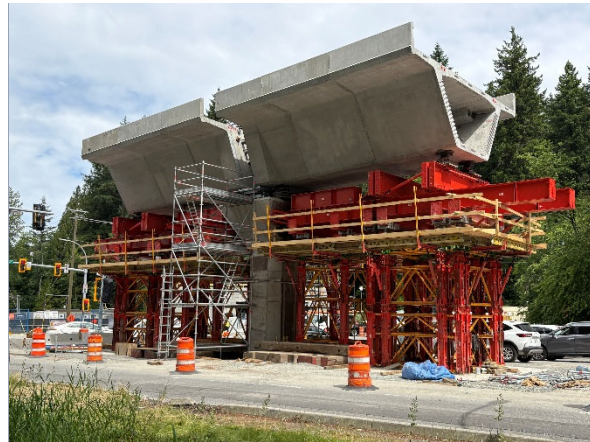
Figure 4: Guideway segments that have been placed by cranes at 96 Avenue and Fraser Highway.
