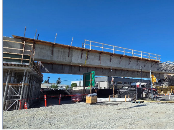
Figure 2: Precast concrete beam installed over 203 Street in Langley City.
