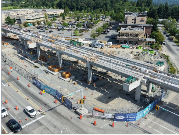
Figure 1: Bakerview-166 Street Station construction.
