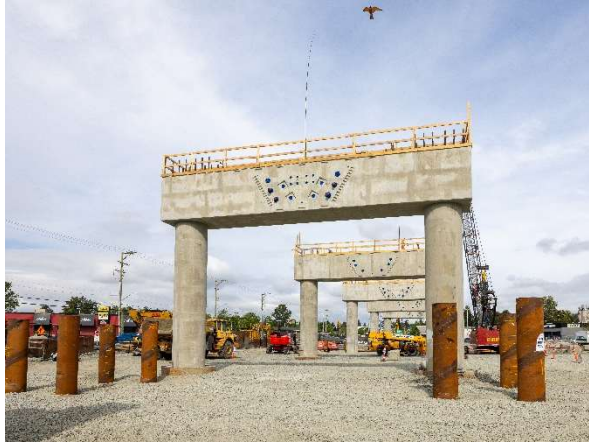
Figure 1: Willowbrook Station guideway columns and bents, and installed station piles.
