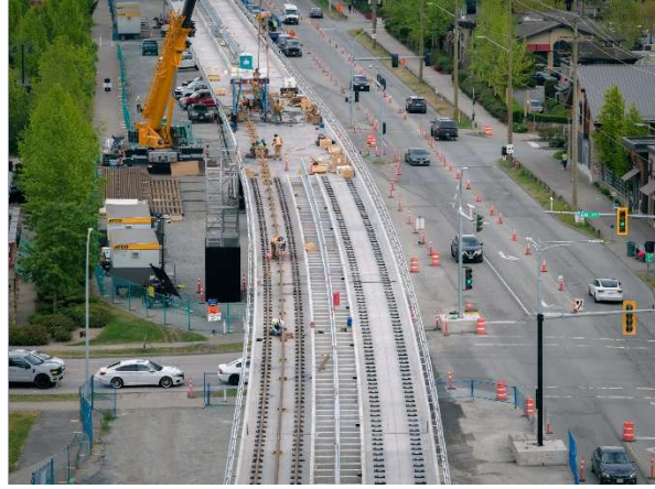
Figure 2: Crews installing rail on the guideway in Clayton near 68 Avenue.
