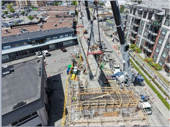
Figure 3: A concrete beam is lifted in place for a guideway span on Industrial Avenue, just west of Langley City Centre Station.
