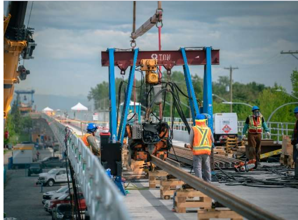
Figure 4: Workers welding running rail pieces together.
