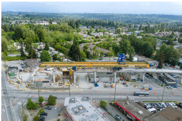
The Fleetwood Flyer building the guideway through the future Fleetwood Station.
