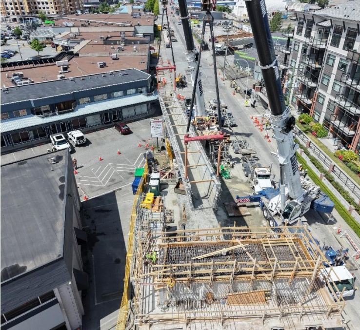
Lifting a guideway beam on Industrial Avenue.
