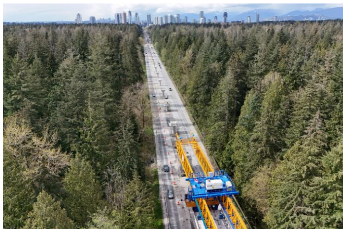
The Surrey Sprinter is working west of 148 Street on Fraser Highway.
