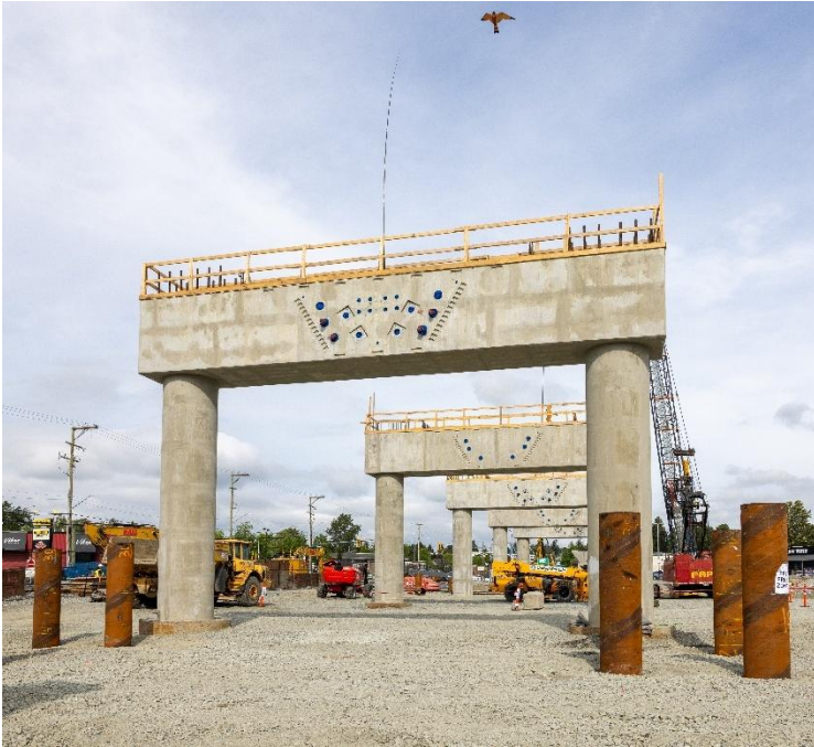
Station foundation piles at Willowbrook Station.
