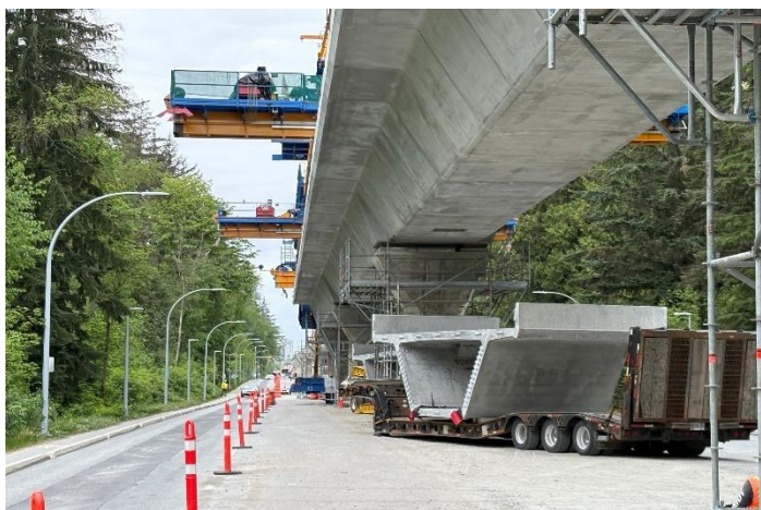
Segment delivery for the Surrey Sprinter.
