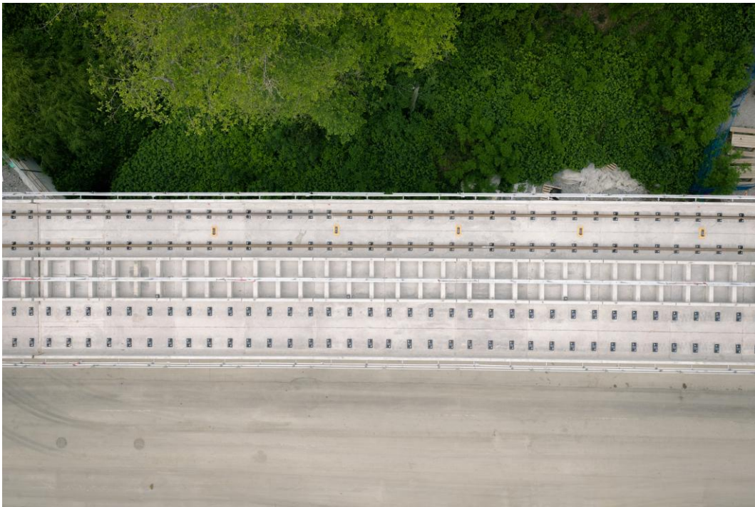
Rail installed on the guideway.
