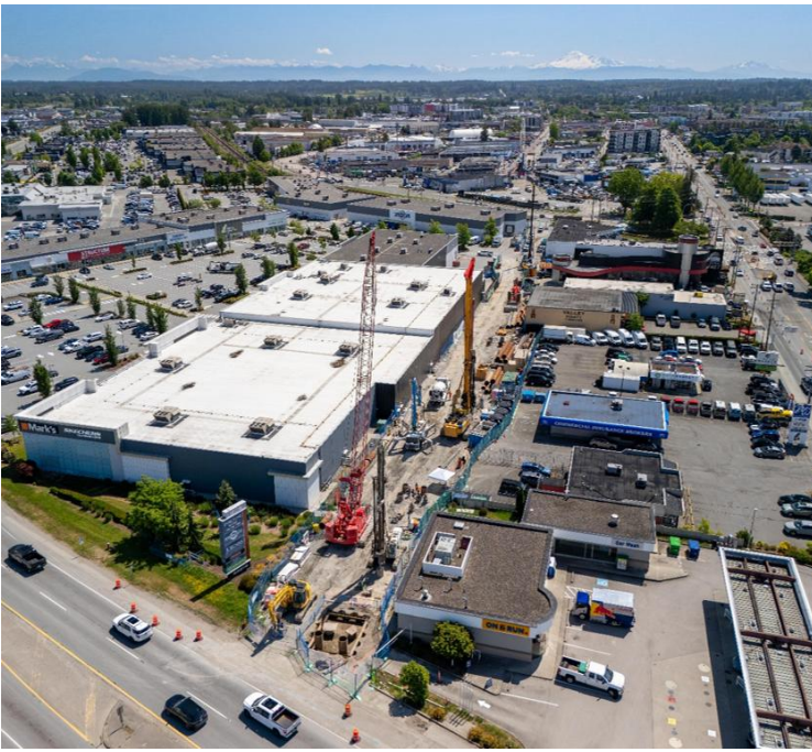
Guideway construction in the laneway east of Highway 10.
