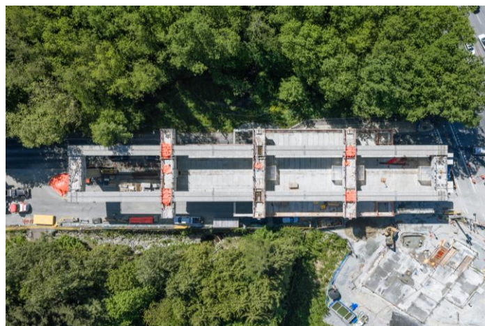
Station construction at the future Green Timbers Station.
