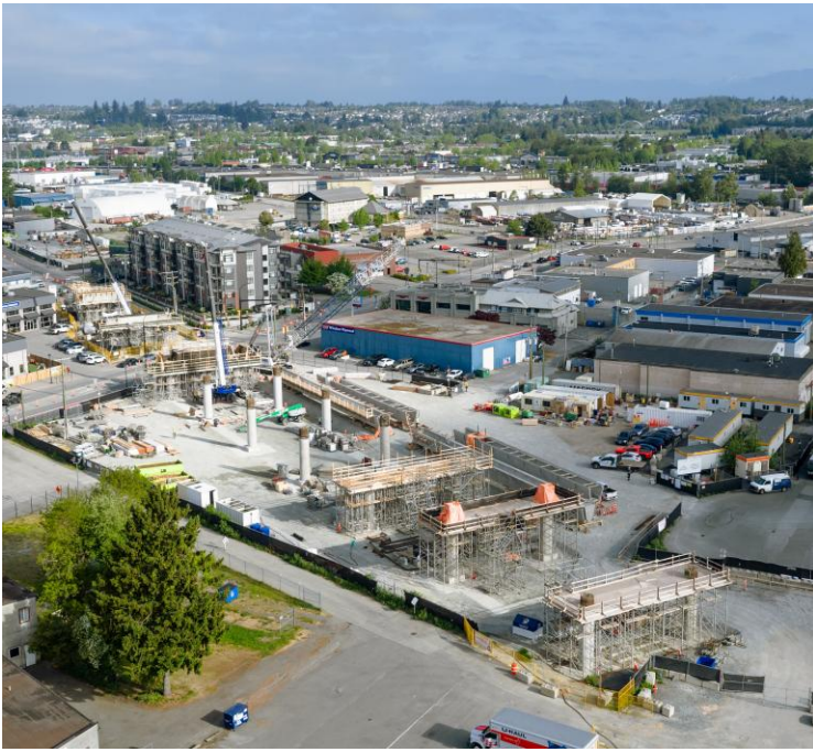
Construction at the Langley City Centre Station.
