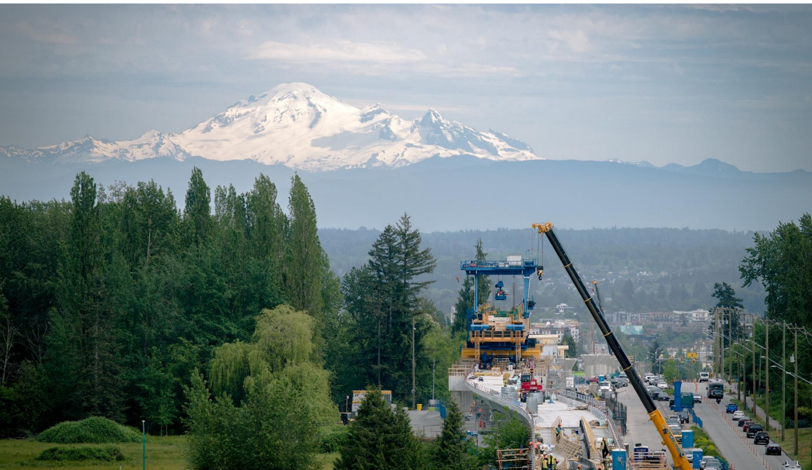
Langley Launcher building the guideway at future Clayton Station.
