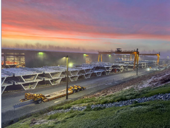
Figure 1: Precast Concrete Facility where guideway segments are produced and stored.
