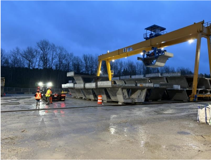
Guideway segments are loaded onto a truck for transport.
