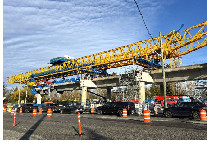
Figure 2: The Clayton Clipper launching gantry near Hillcrest – 184 Street Station.
