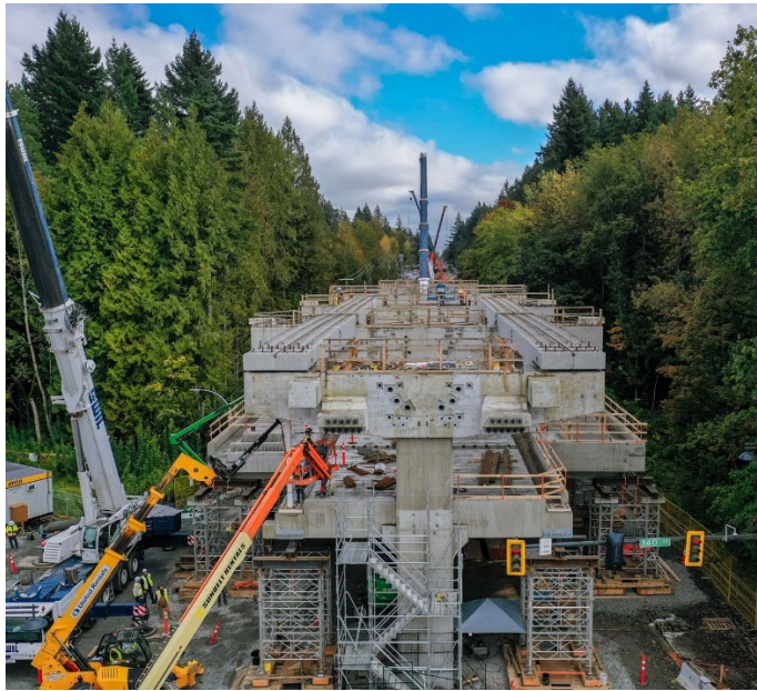
Figure 3: Construction of Green Timbers Station. Crews have installed concrete beams which serve as the main structural support for the mezzanine.
