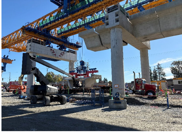
Figure 1: A segment being lifted into place by the Surrey Sprinter launching gantry near 152 Street Station.
