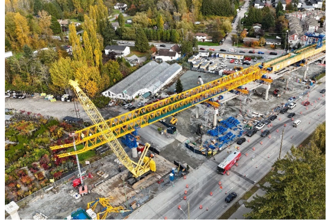
Figure 2: The Langley Launcher and Clayton Clipper launching gantries side-by-side at Hillcrest-184 Street Station.
