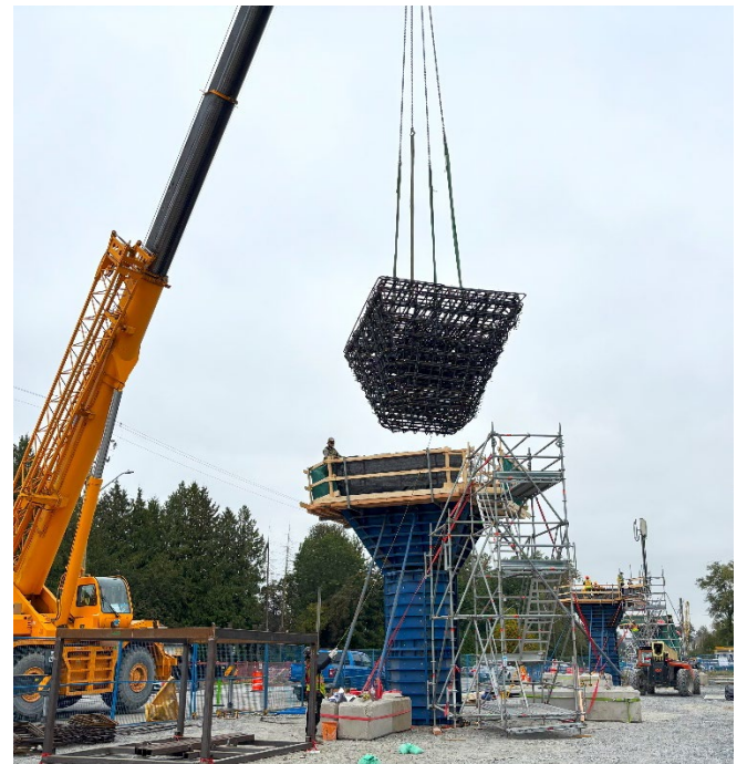
Figure 4: Tulip column construction.
