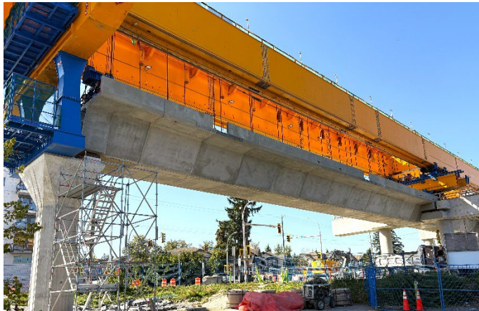
Figure 1: The first completed span outside of a station site installed by the Fleetwood Flyer launching gantry.
