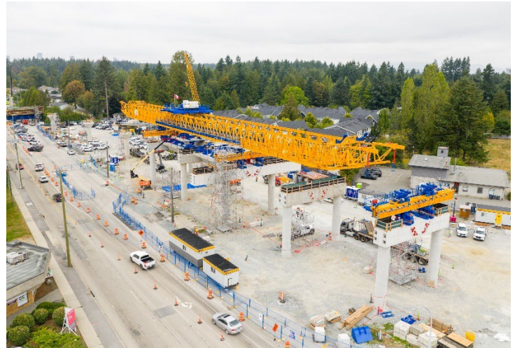
The Surrey Sprinter installing spans at 152 Street Station.
