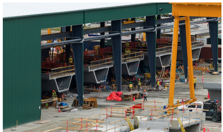
Guideway segments at the precast concrete facility.
