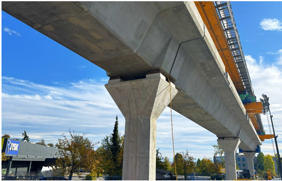
Completed spans east of Bakerview-166 Street Station.
