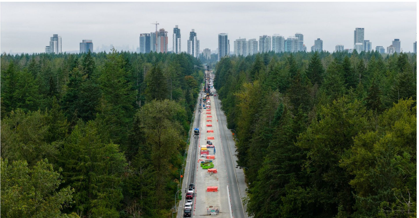
Single lane traffic near Green Timbers Urban Forest during construction.
