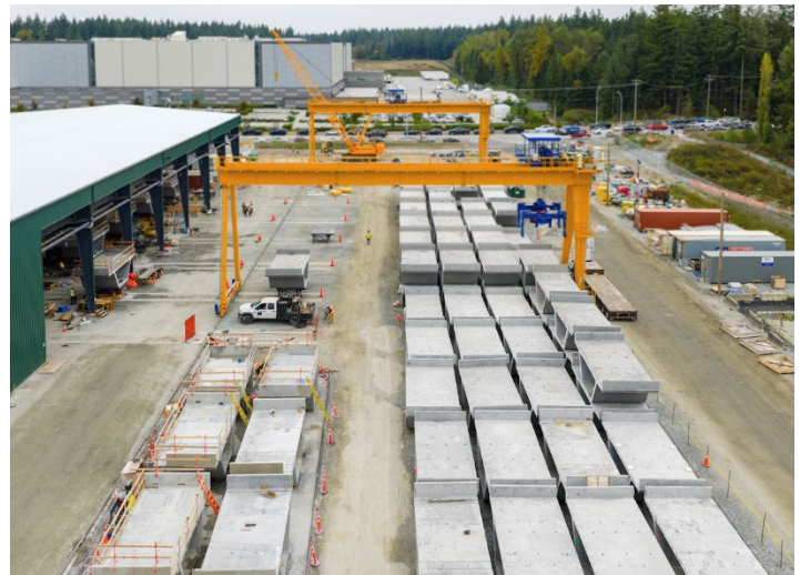
Guideway segments at the precast concrete facility.
