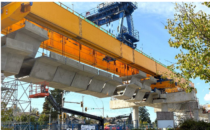
The Fleetwood Flyer constructing spans just east of Bakerview-166 Street Station.
