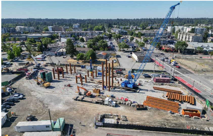
Foundation construction at Langley City Centre Station.
