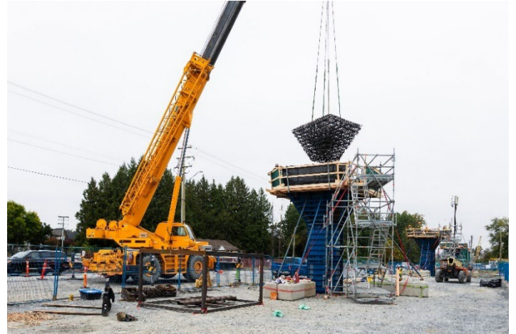
Tulip columns along Fraser Highway.
