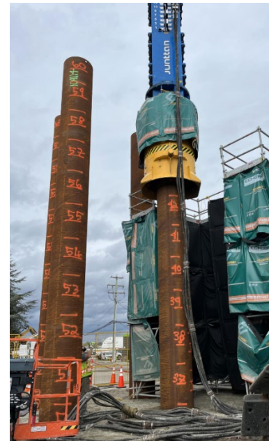
Elevated guideway foundation construction on Industrial Avenue.
