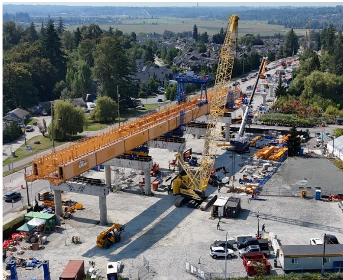
Figure 1: The Fleetwood Flyer launching gantry continuing to lift and install segments at Bakerview-166 Street Station.
