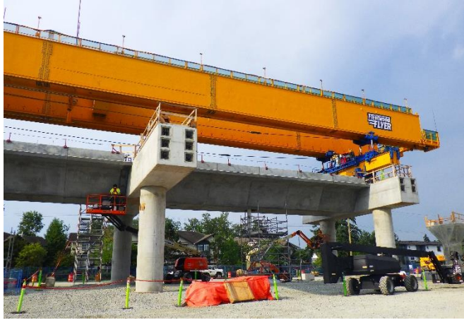
Figure 1: The Fleetwood Flyer launching gantry continuing to lift and install segments at Bakerview-166 Street Station.
