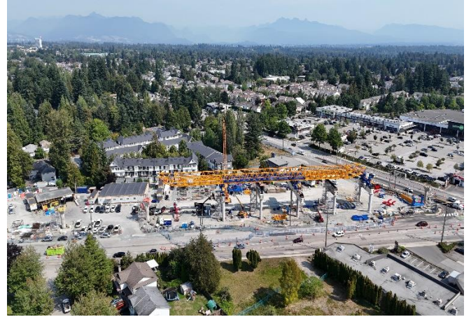
Figure 2: Aerial photo of the Surrey Sprinter launching gantry being assembled at 152 Street Station.
