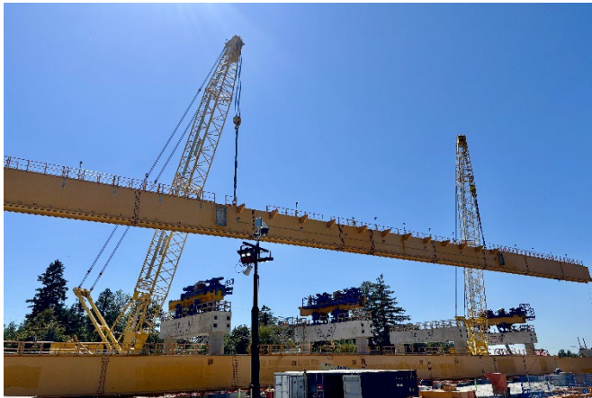
Figure 1: The Fleetwood Flyer launching gantry lifting and installing guideway segments at Bakerview-166 Street Station.
