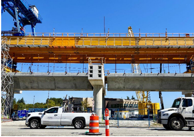
Figure 1: The Fleetwood Flyer launching gantry lifting and installing guideway segments at Bakerview-166 Street Station.
