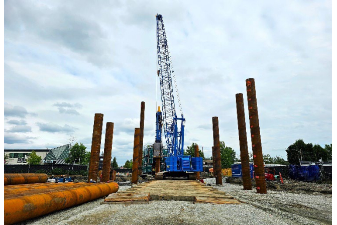
Figure 2: Piles being installed into the ground at the site of Langley City Centre Station.
