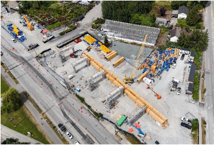
Launching gantry parts at Hillcrest-184 Street Station.
