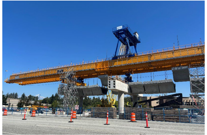
The Fleetwood Flyer lifting guideway segments.
