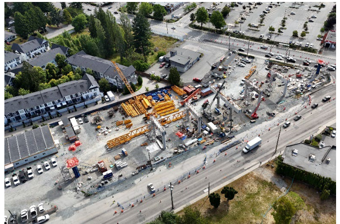
Launching gantry being assembled at 152 Street Station.
