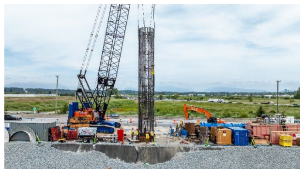
Rebar cage installation as part of foundation construction near Fraser Highway and Highway 15.
