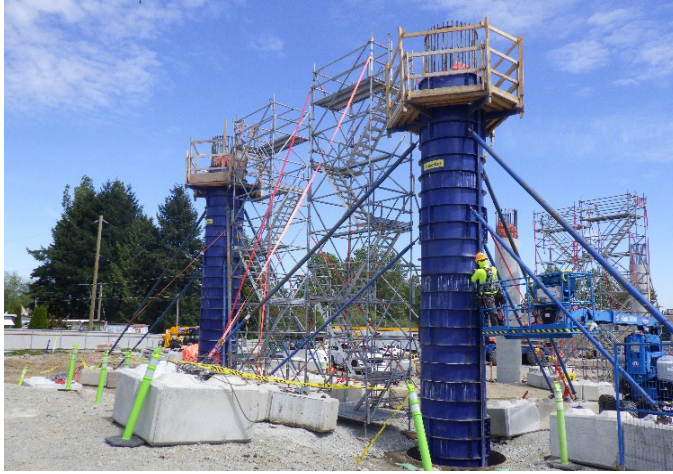
Figure 1: Formwork installation for columns at the future Fleetwood Station.
