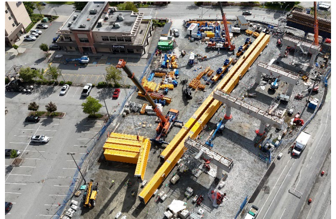
Figure 4: Aerial shot of Bakerview-166 Street Station with launching gantry pieces ready to be assembled.
