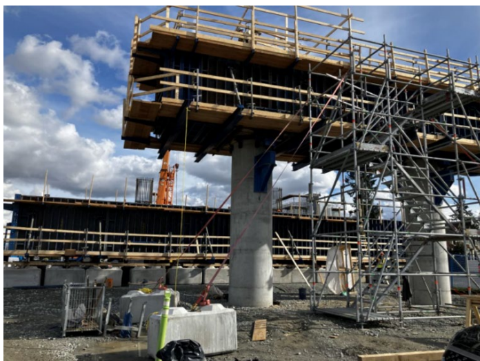
Guideway pier cap construction underway at Bakerview-166 Street Station.
