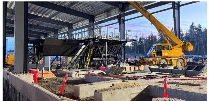
Work within the steel building to assemble one of the molds for the guideway.
