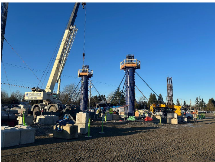
Guideway pier installation underway at 152 Street Station.
