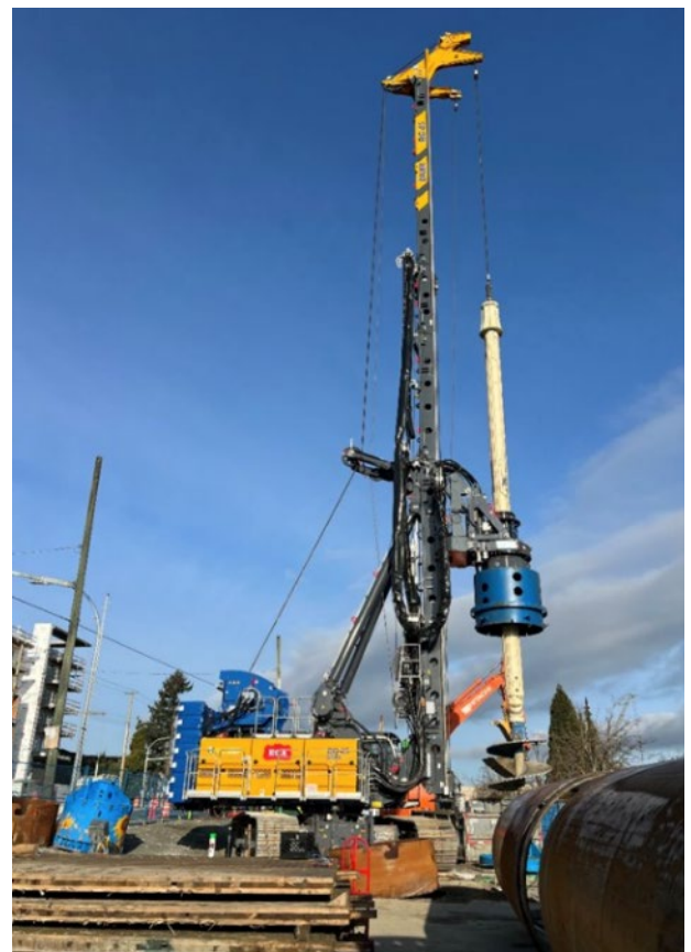
Foundation construction, including drilled piles, is ongoing at Bakerview- 166 Street Station.
