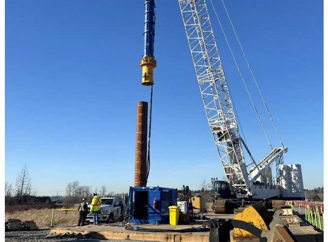
Figure 2: Driven piling underway near the intersection of Fraser Highway and 176 Street (Highway 15).
