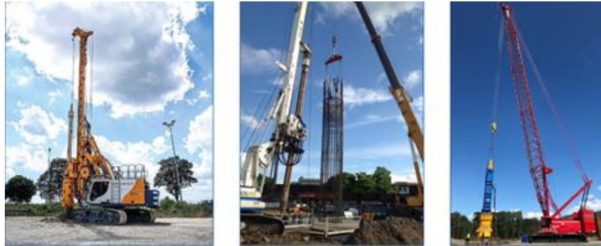
Fig: Mobile cranes and drill rigs will be used for foundation installation.
