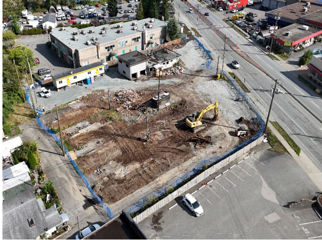
Figure 1 - Demolition activities completed at 16039 Fraser Highway to accommodate SkyTrain infrastructure.
