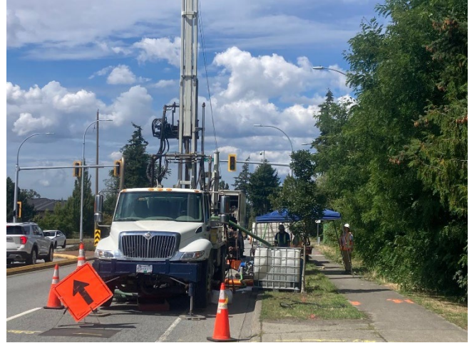
Figure 2 - Borehole investigative works ongoing at several locations along the Fraser Highway.
