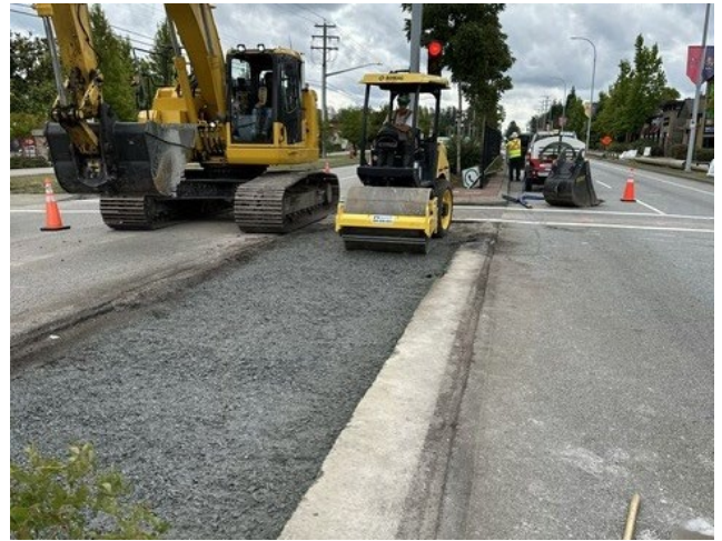
Figure 4 - Median removal activities ongoing at multiple locations along the Fraser Highway.
