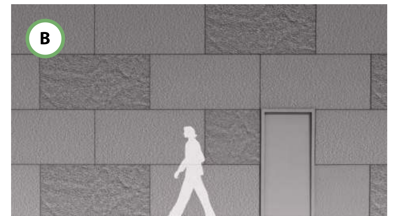
Station specific design on exterior cladding panels
