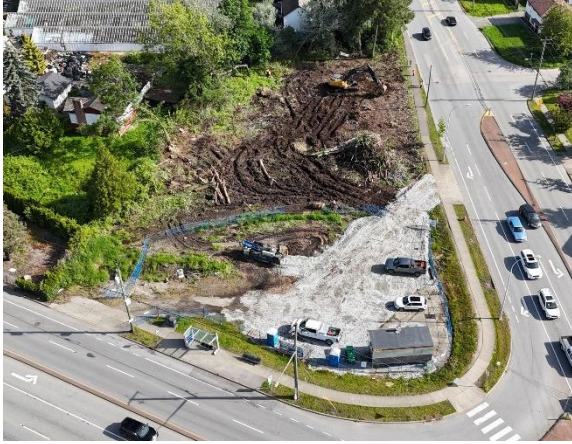
Figure 1: Aerial view of site preparation at Hillcrest-184 Street Station.
