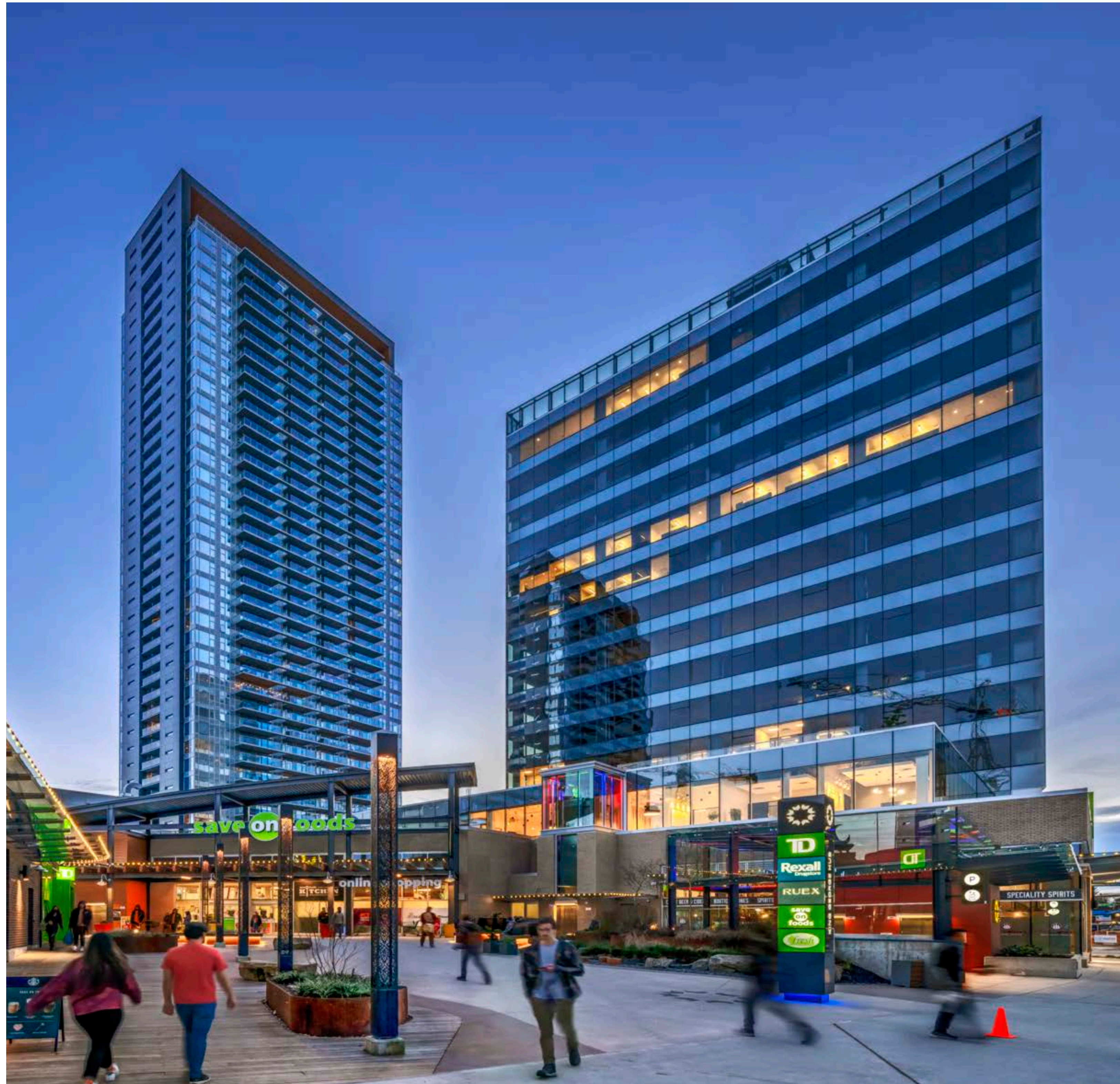
*Photo Courtesy of PCI Developments
