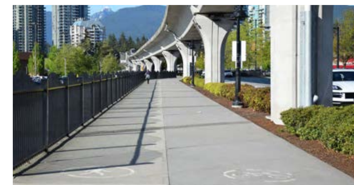
Combination of pavement finishes defines use
